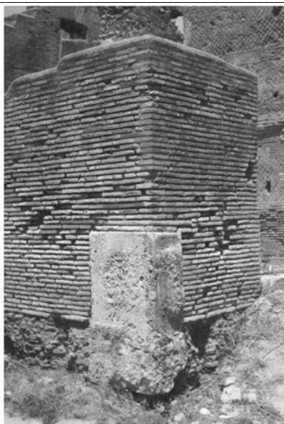
The image above, showing a cornerstone, is from the ancient Roman city of Ostia. Here the cornerstones seemed to have also marked the property boundaries for the houses (called insulae).
