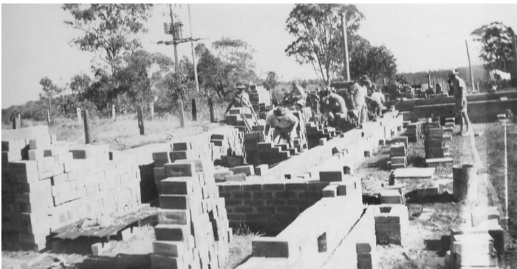
Brick construction underway
